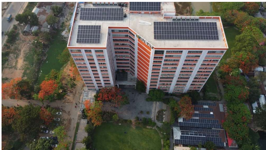
A 234 KW solar panel installed at the roof top of the campus building
