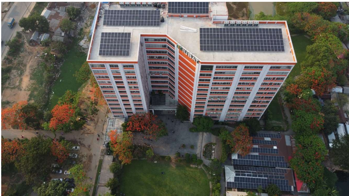
A 234 KW solar panel installed at the roof top of the campus building
